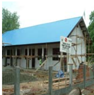
Primary School construction in Aceh.
