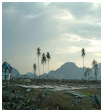
Destruction caused by the Tsunami in Indonesia.
