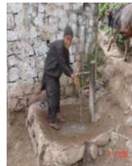
Islamic Relief Worldwide installed water pump in Bagh, Pakistan.
